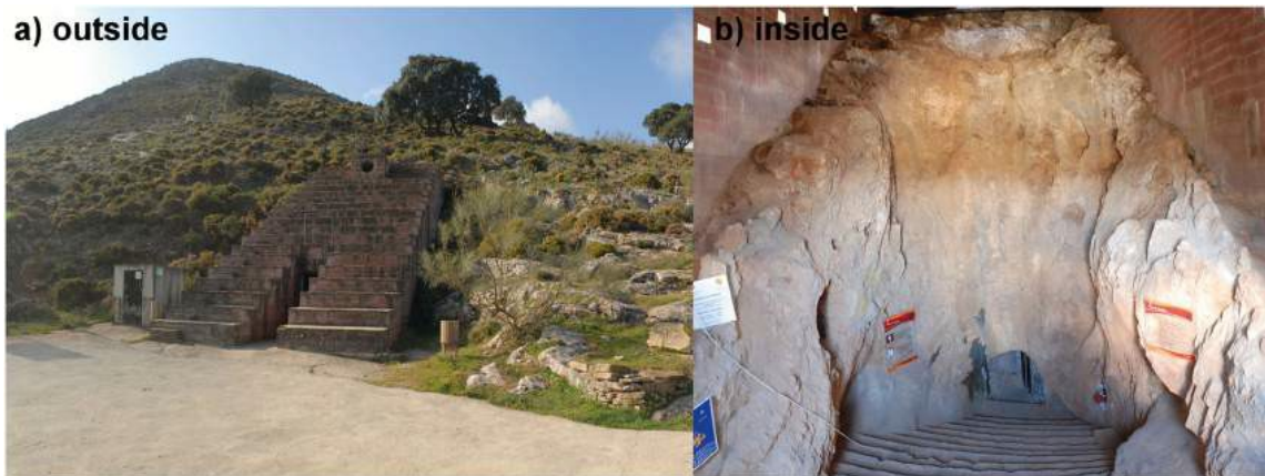
Figure 6. Panoramic picture of the entrance area with the building that was virtually removed together with the inside door to conduct the lighting simulation. This figure is available in colour online at wileyonlinelibrary.com/journal/arp
