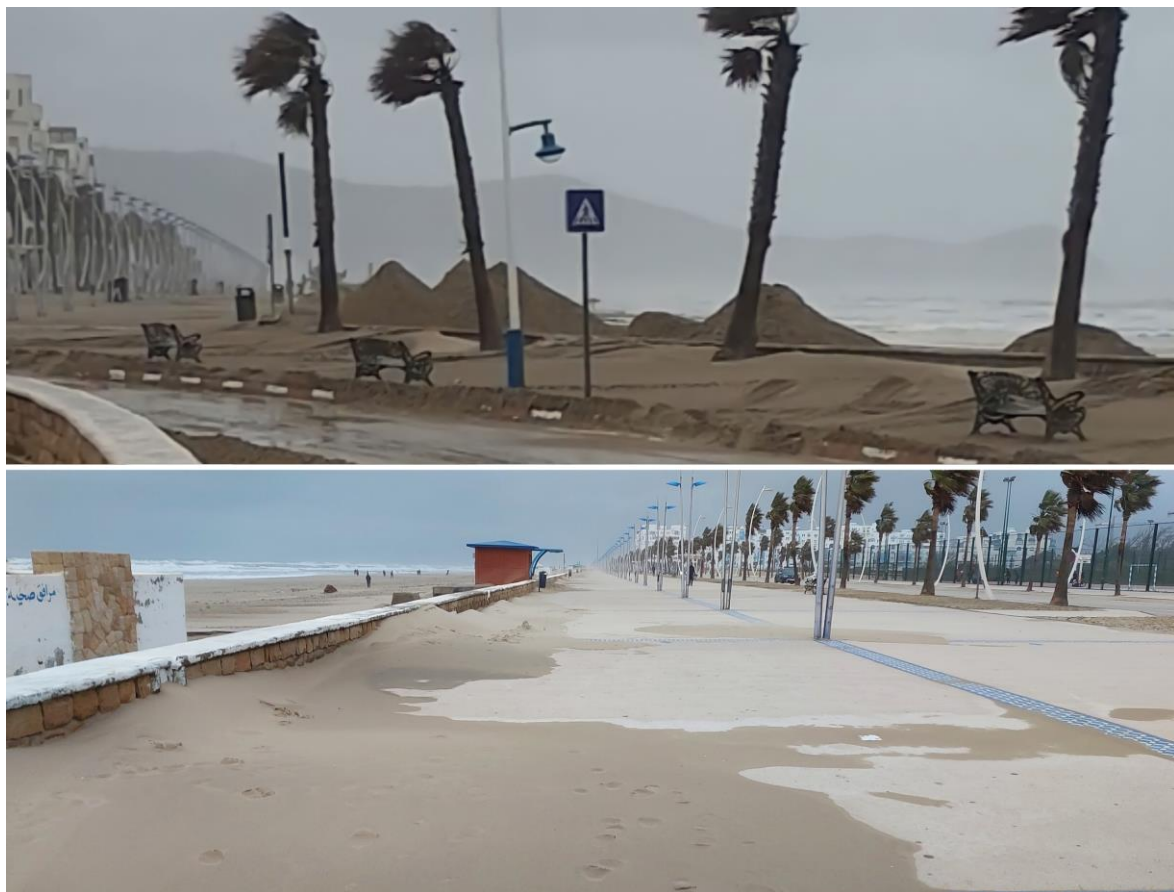
Figure 8. Silting of the tourist promenade and coastal road backing the beach of Martil.
